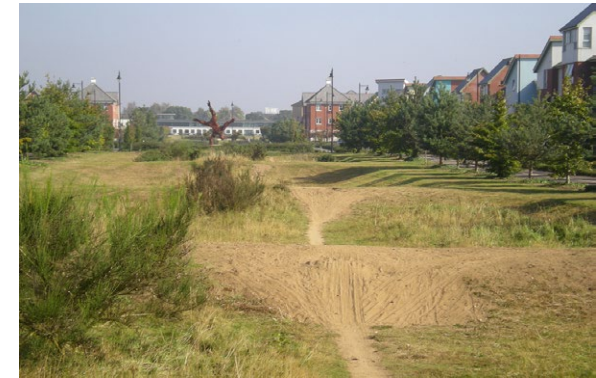
SuDS infiltration basins have been integrated with highways at Ravenswood in Ipswich. The scheme is estimated to have saved over £600,000 in the long term (Ipswich Borough Council, 2011)
