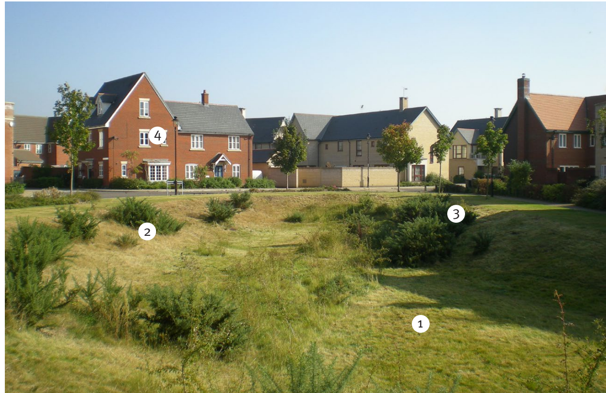
Infiltration basin at Ravenswood
