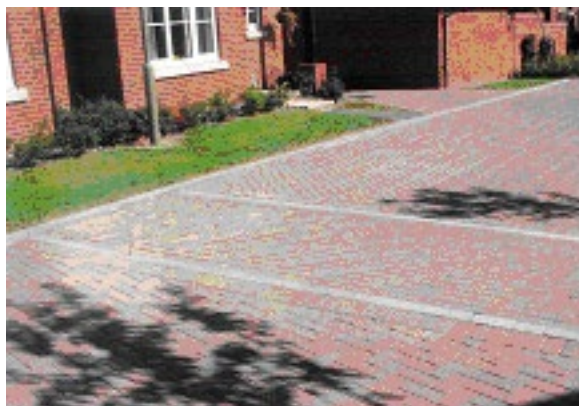
SuDS service crossing
