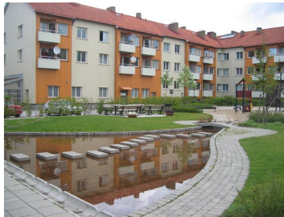
The SuDS ponds at Augustenborg in Malmo are integral features of the courtyards
