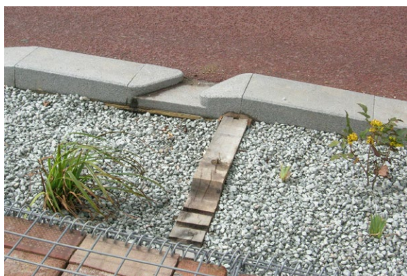
SuDS Highway detail, Ashford, Kent
