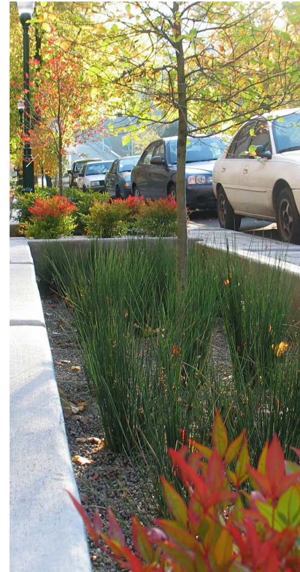
Bio-retention planters, Portland, Oregon, USA
