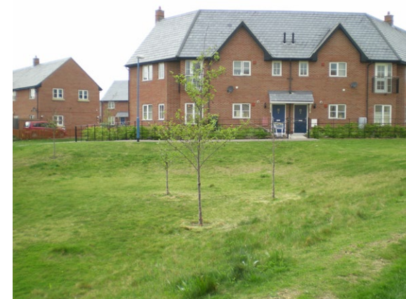
Detention basin at 'Lamb Drove', Cambourne
