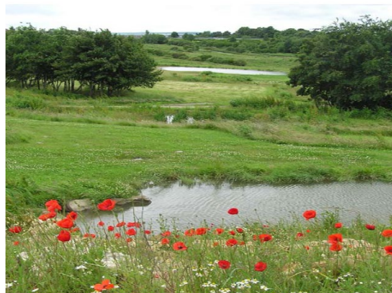
Basins and swales carved from the slopes at Manor Park in Sheffield store and treat run-off from residential areas (above) and are used for events space when dry (below) (Sheffield City Council, 2011)
