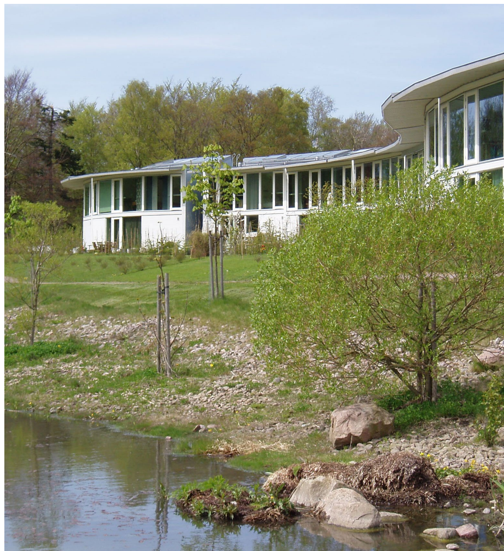
Wetlands store/treat run off at residential development, EOS Bostadsrättsförening, Sweden
